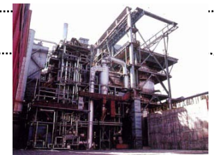
Coke dry quenching equipment (CDQ)
