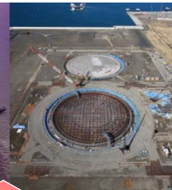
(Naoetsu LNG Receiving Terminal : Under construction)
