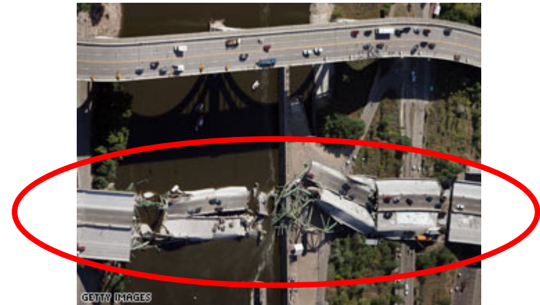
The Interstate 35W bridge collapsed into the Mississippi River during rush hour in 2007.
