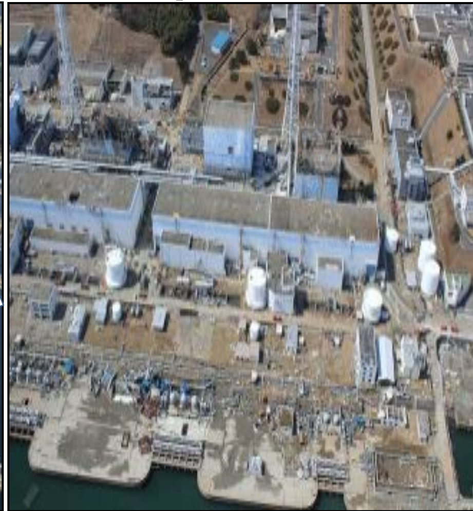
After the Earthquake and Tsunamis
